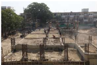
Construction of Rabia Rasheed Soorty building in progress.
