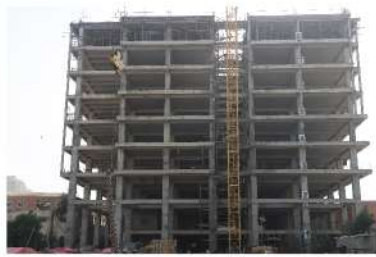
Construction of Medical Tower, comprising 8 Floors is under construction.
