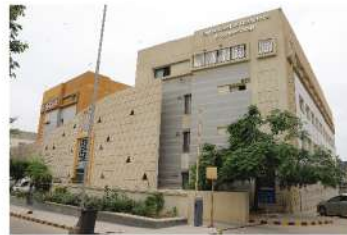
Renovation of Gyne & Emergency wards.
