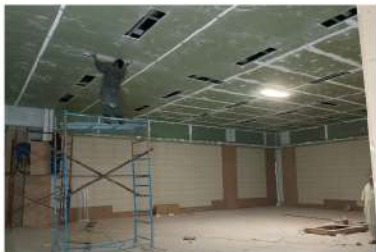
Construction of Lecture Hall at Surgical Complex is in progress.
